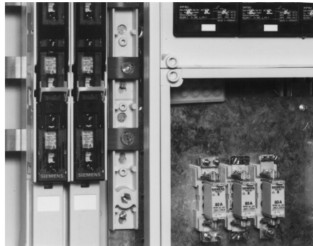
LV HRC fuse links in fuse bases and in-line fuse switch-disconnectors in a floor-mounted SIKUS distribution board
